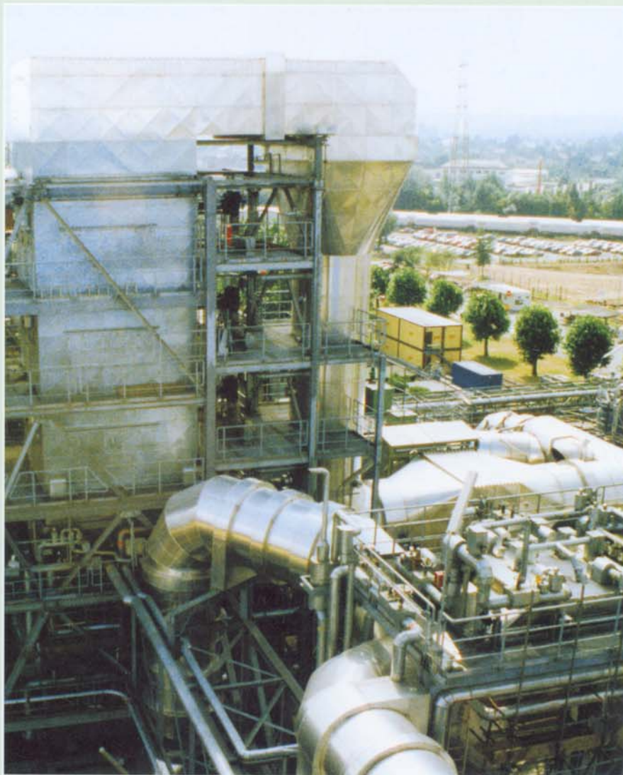
Katalysatorsystem (SCR)
